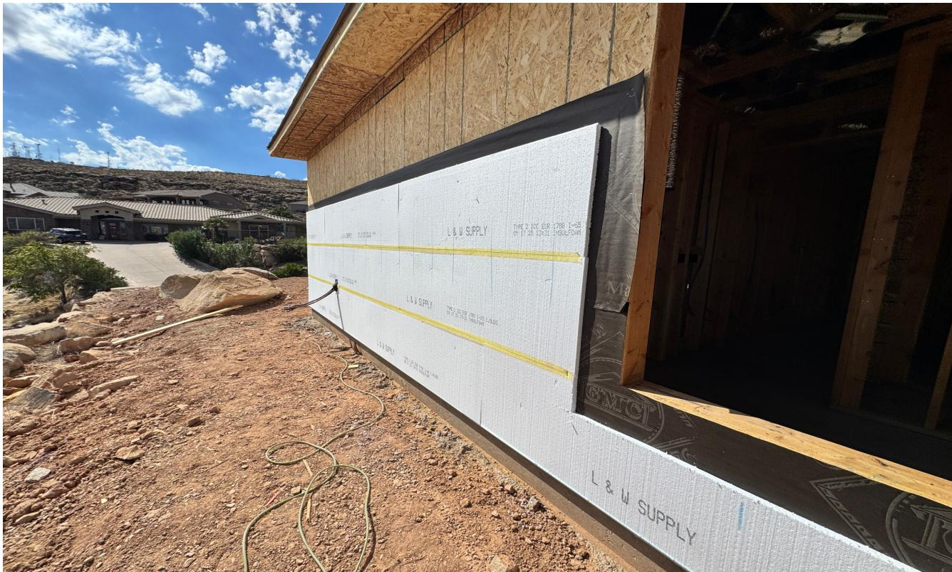
Exterior foam insulation plays a critical role in blocking radiant heat from sun. By wrapping the home in continuous insulation, we minimize thermal bridging and help maintain stable indoor temperatures.
